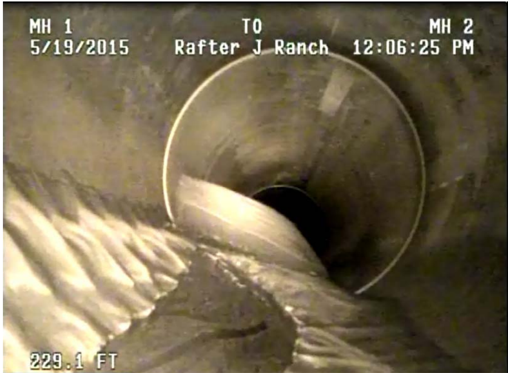
Photograph 7: View of apparent sand mound at upstream end of clear well pipe.
