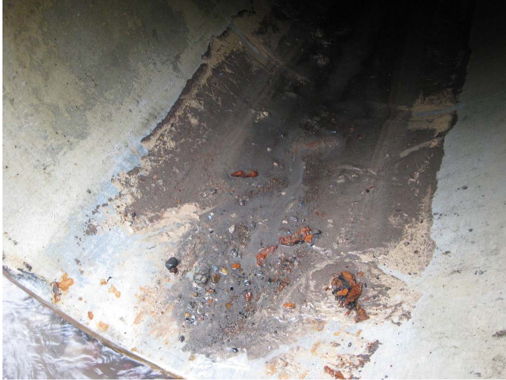
Photograph 3: View of fines, sediment and other debris inside downstream end of clear well pipe.
