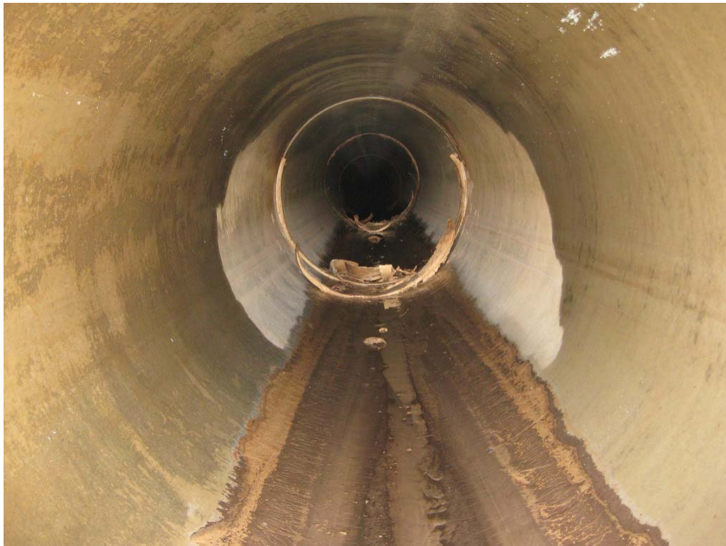
Photograph 4: View inside clear well pipe. Note mortar/grout material at pipe seam.
