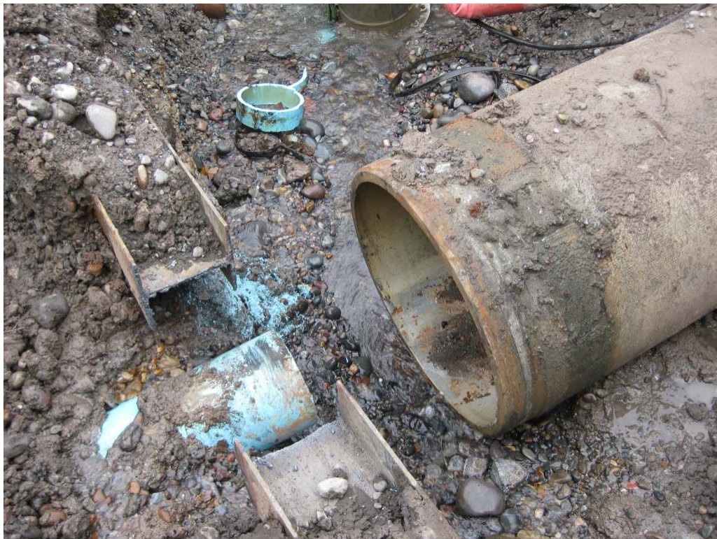
Photograph 2: View of clear well cement pipe with steel end cap removed.
