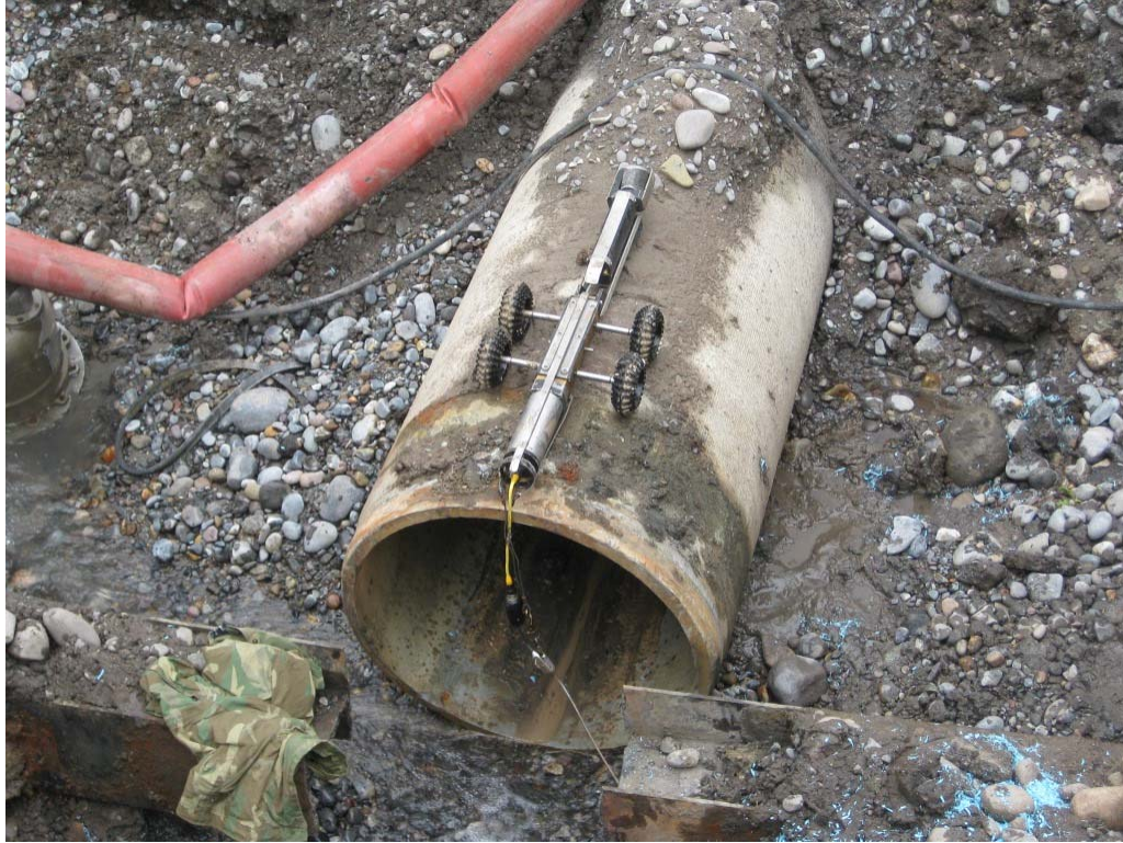
Photograph 5: View of remote controlled camera vehicle.
