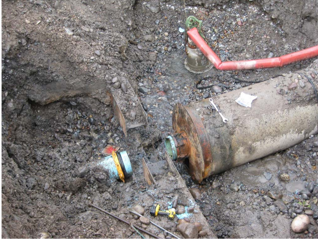
Photograph 1: View of clear well cement pipe with steel end cap intact.
