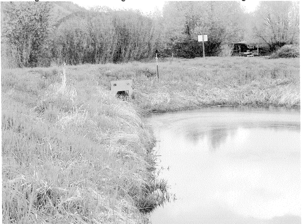
Looking southeast at wetland outlet culvert.
